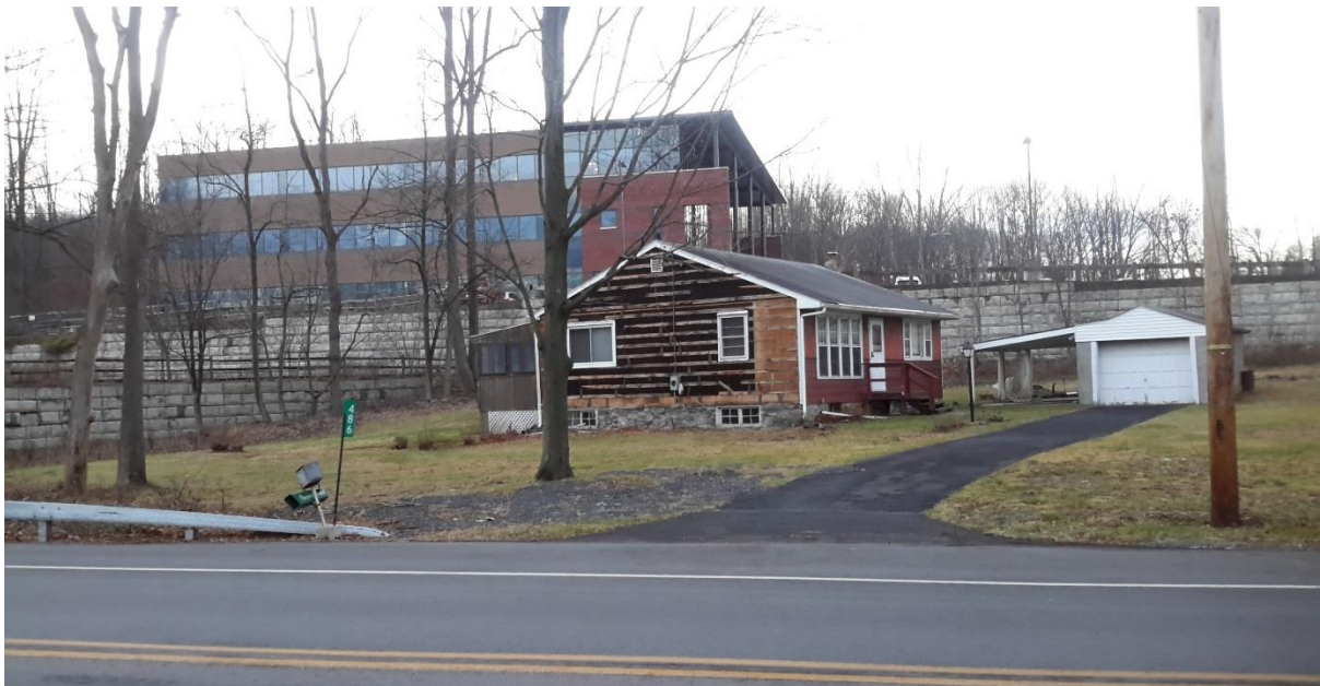
486 East Brown Street East Stroudsburg, Pennsylvania
