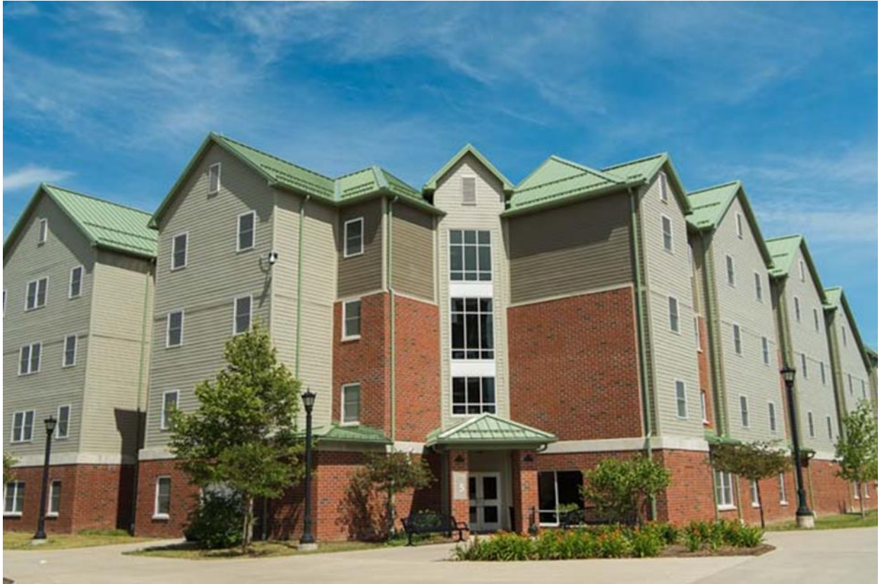
Typical Highlands Residence Hall
