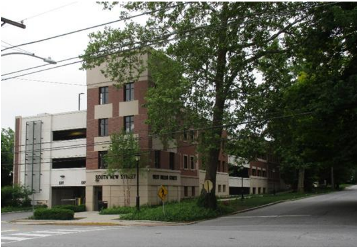
New Street Garage, West Chester University of Pennsylvania
