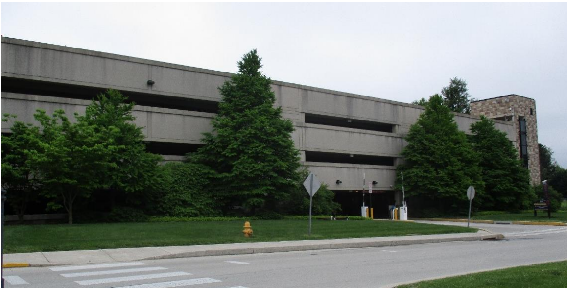
Matlack Street Garage, West Chester University of Pennsylvania
