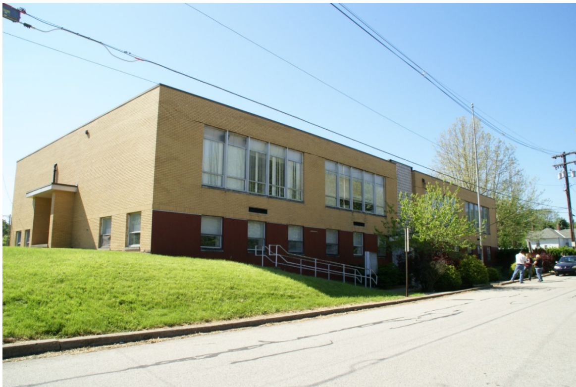
Main Office Building 750 Orchard Street, California, Pennsylvania
