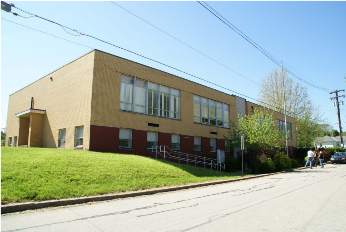
Main Office Building 750 Orchard Street, California, Pennsylvania
