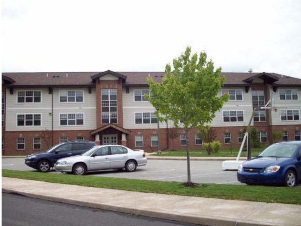
Punxsutawney Regional Campus, Student Residential Facility View from Southwest
