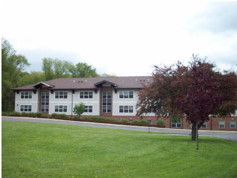
Punxsutawney Regional Campus, Student Residential Facility View from West
