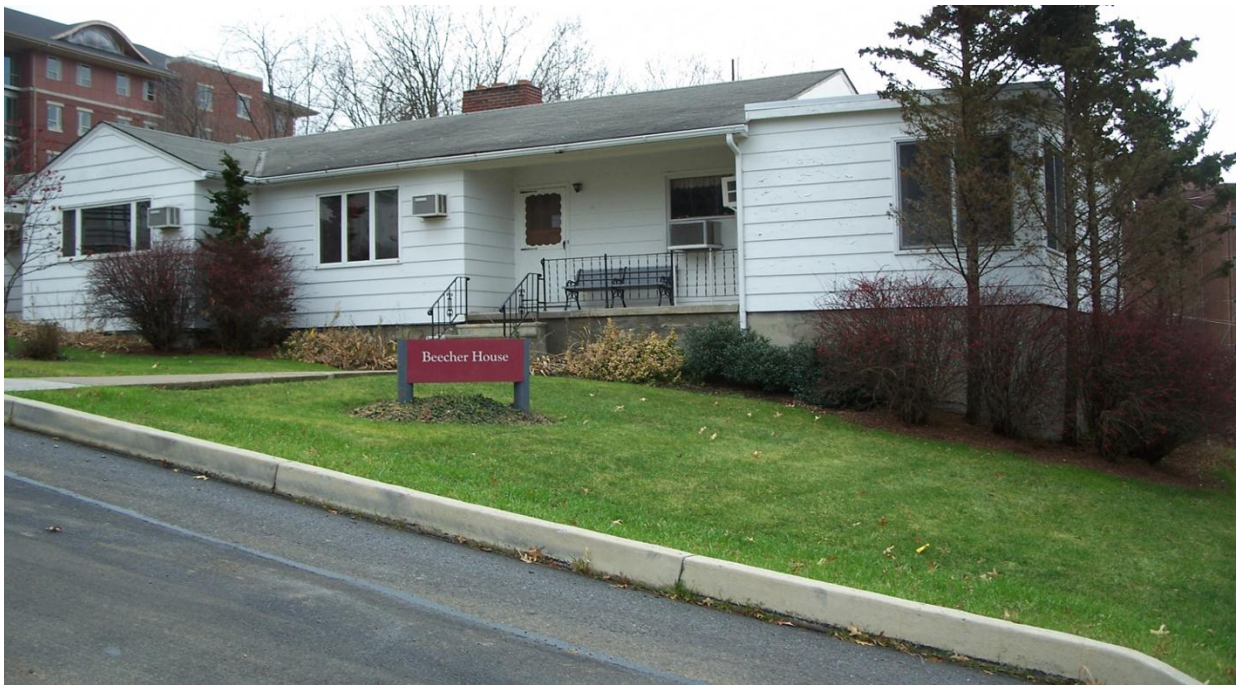
Beecher House Mansfield University of Pennsylvania
