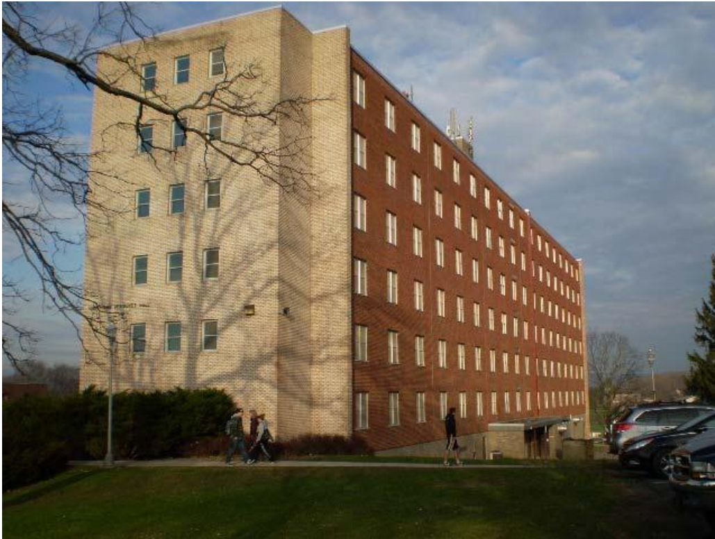
Hawthorn Residence Hall East Stroudsburg University of Pennsylvania
