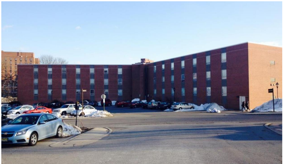
Hull Hall Millersville University of Pennsylvania
