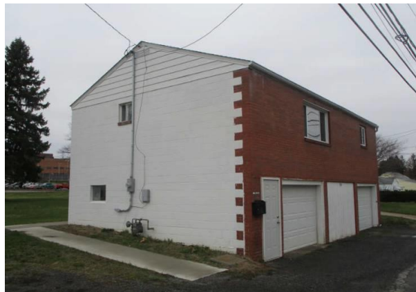
Vacant Lot, Garage and Apartments at 915 Corbett Street and 177 Greenville Avenue
