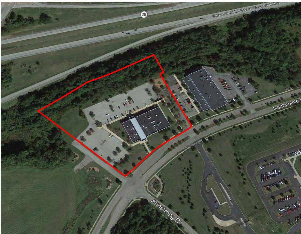
IUP Northpointe 167 Northpointe Boulevard, Freeport, Armstrong County, Pennsylvania, 16229
