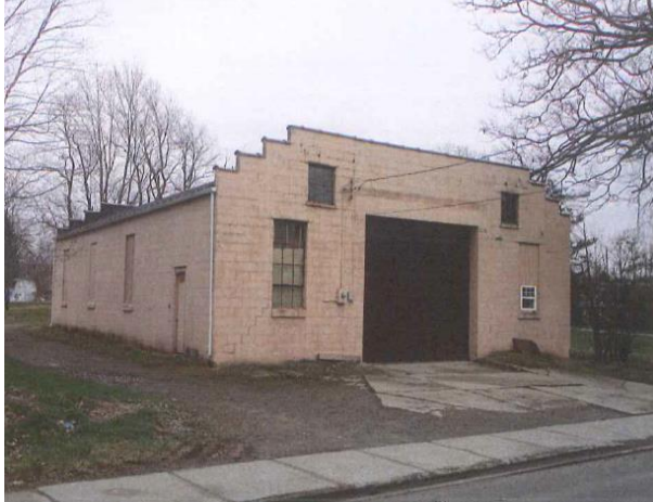
Vacant Lot and Warehouse at 215, 221–221½ Greenville Avenue, Clarion, Pennsylvania
