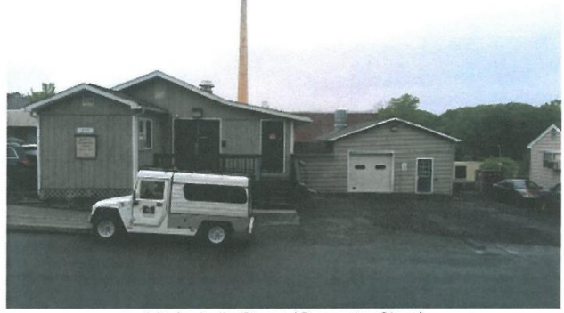
111 Isabelle Street (Carpenter Shop)
